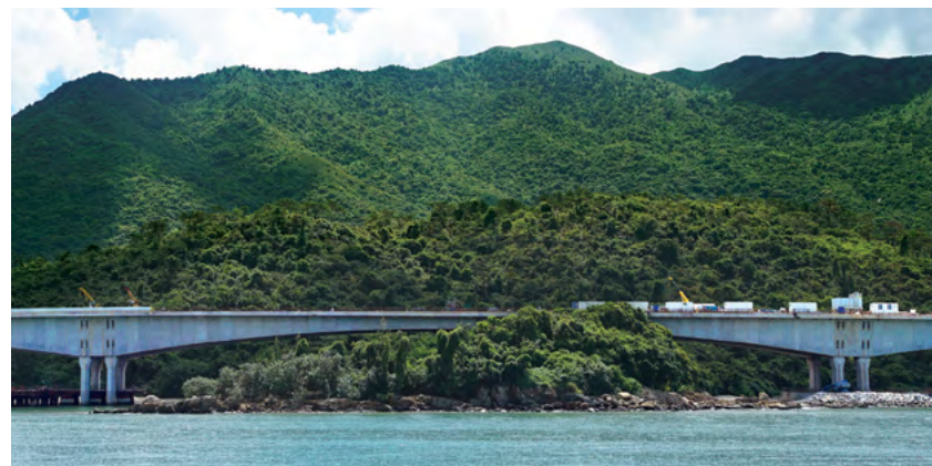
The world's LARGEST span of a pre-cast segmental balanced cantilever bridge span at 180m 大橋當中180米跨度是全球最長的懸臂分段拼裝式預製橋
