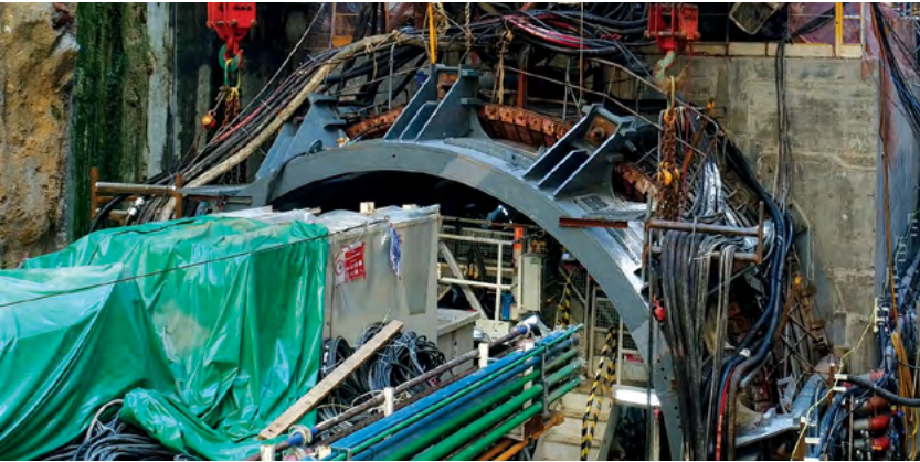
The “starwheel with pre-stressed bars”, together with the 40m-deep peanut shaft, earned us the “Gold Award – Temporary Works Excellence Award 2017 – Civil Engineering Works” 我們憑著「先張預應力星形輪鋼架」及深40米的無橫向支撐環形豎井，於「2017臨時工程卓越大獎」土木工程組別中取得金獎殊榮
