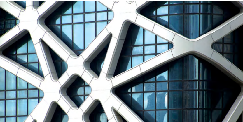
Morpheus – the world’s FIRST free-form exoskeleton high-rise building 摩珀斯是世界上首座採用自由形態外骨骼結構的高樓
