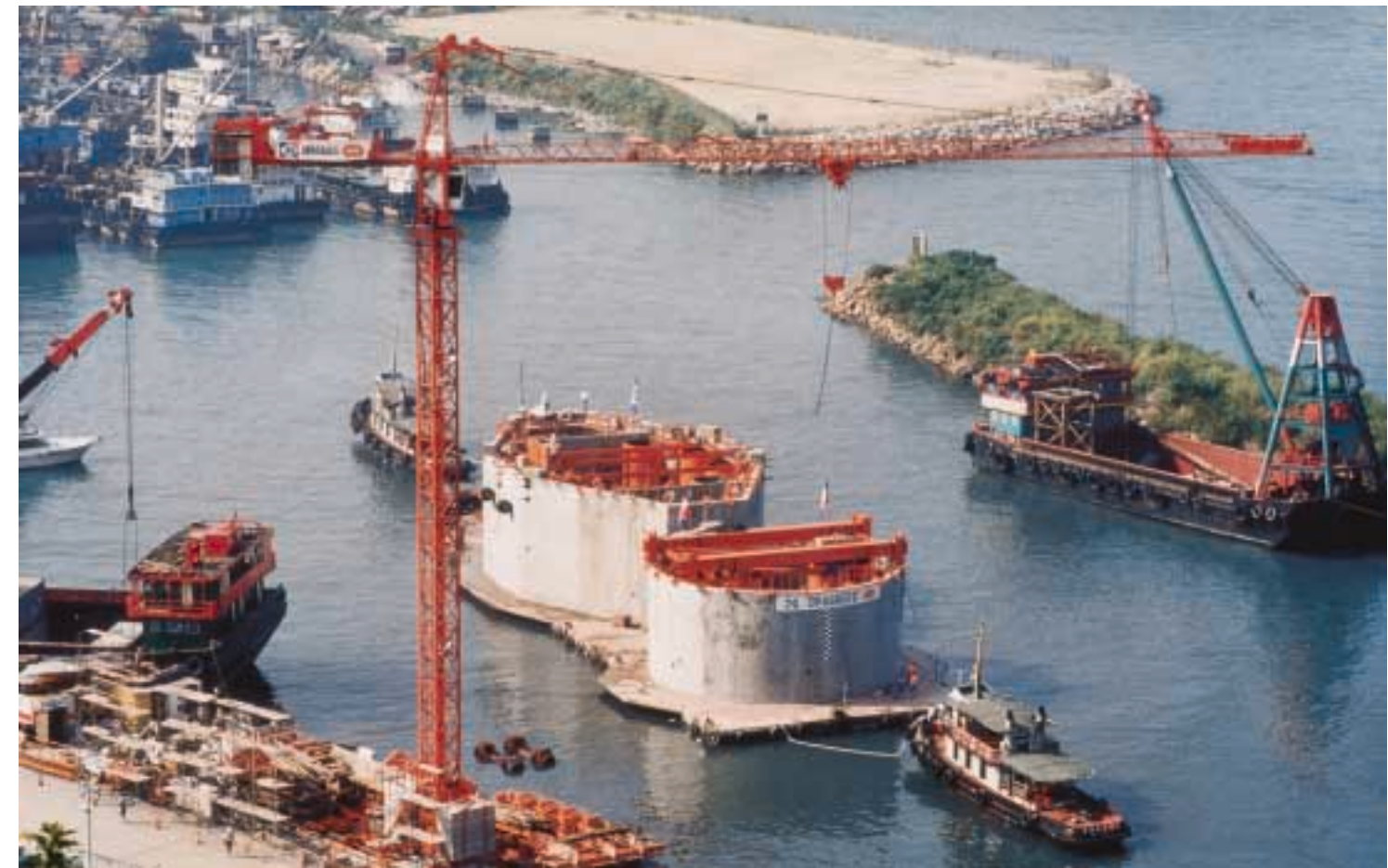
Towing the caissons to the site 沉箱就位
