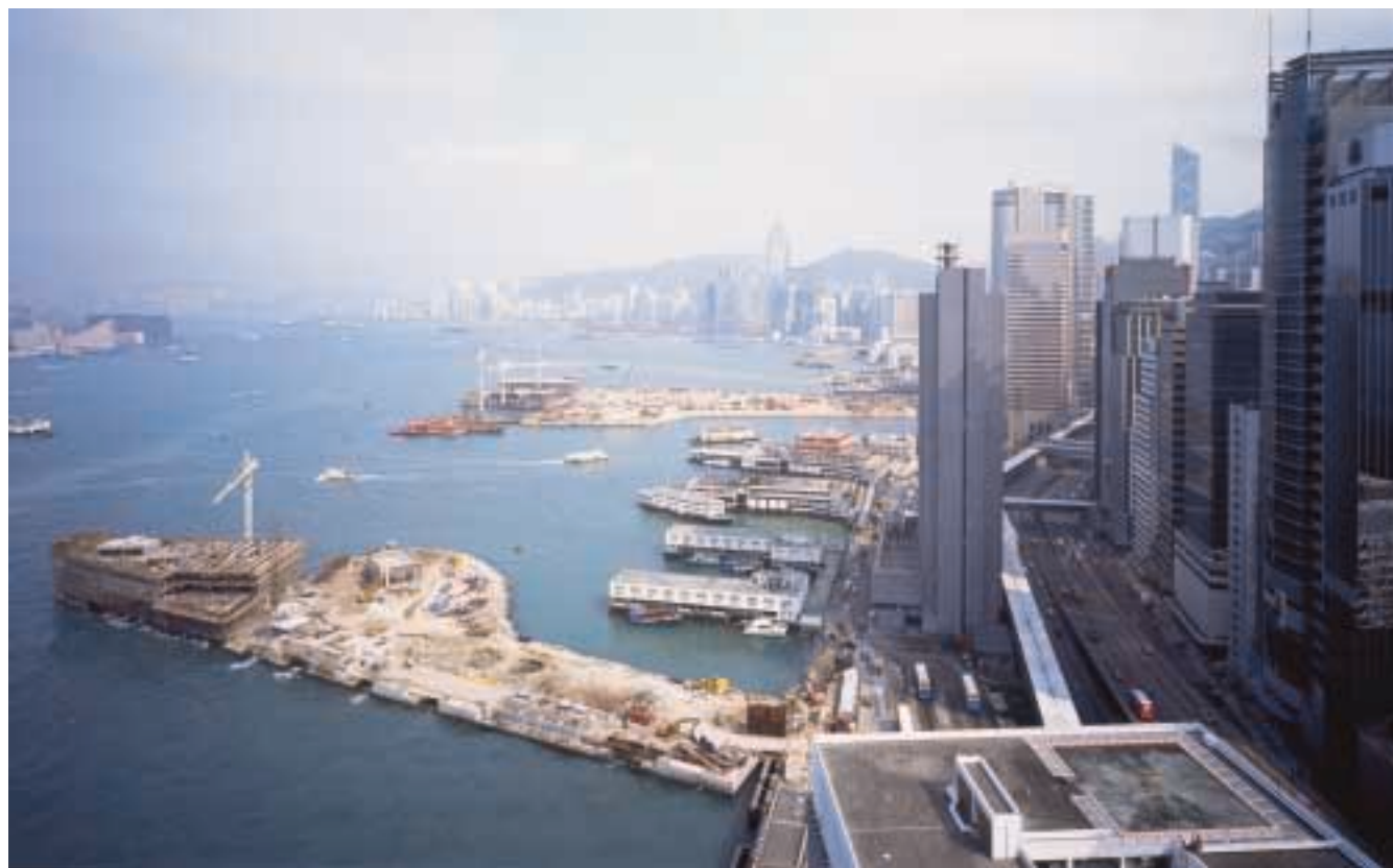
New piers were being constructed while the old piers remained in use 在興建新碼頭的同時，舊碼頭繼續為市民服務
