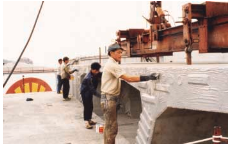
Workers applying extra strength segment glue 工人施加特製強力膠
