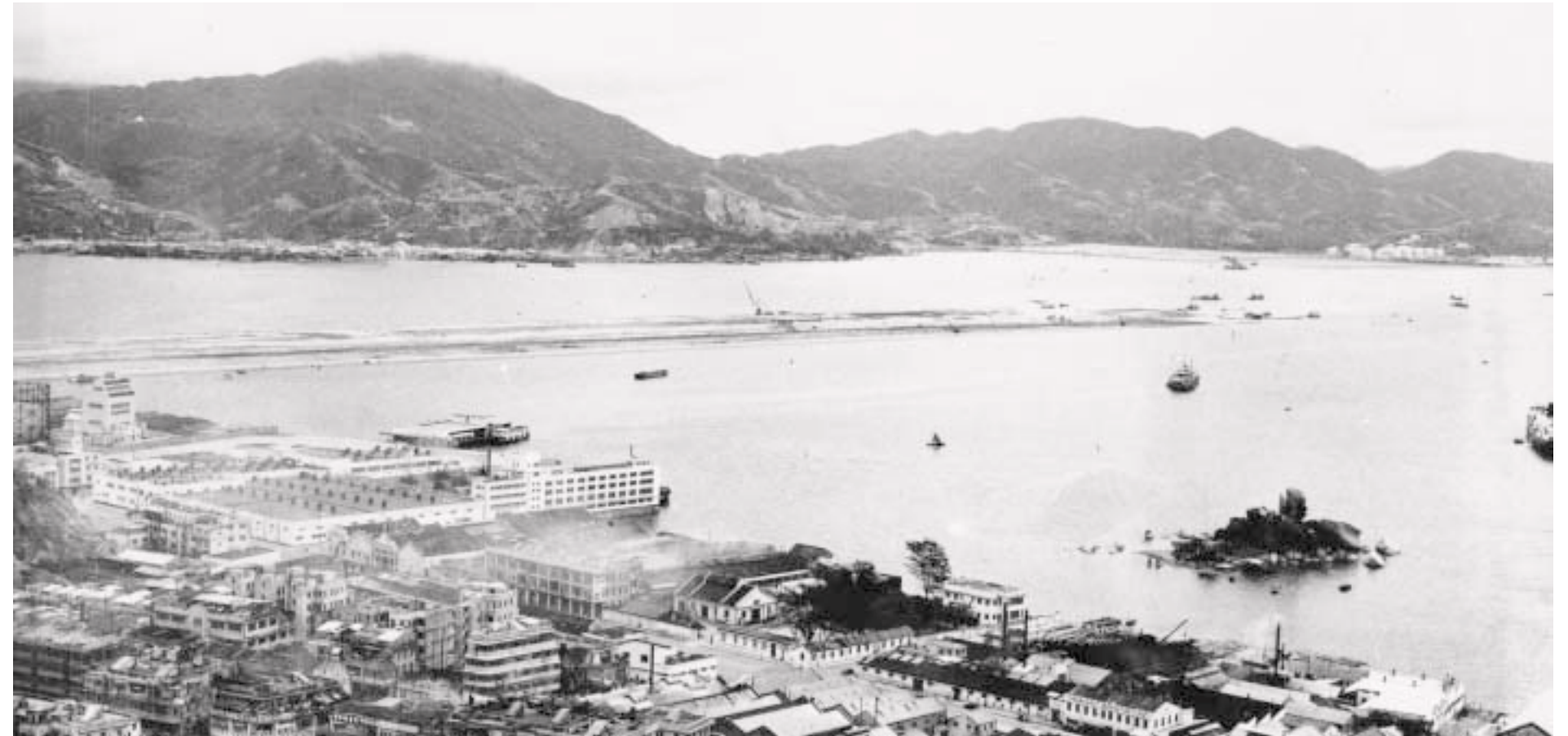
1,850,000 m 3 of mud was dredged from the seabed 由海床挖出 1,850,000 立方米淤泥
