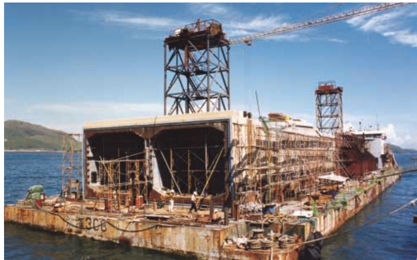
A massive precast tunnel segment, part of the Airport Express, was towed to site 起用躉船，運送機場快綫隧道預製管道
