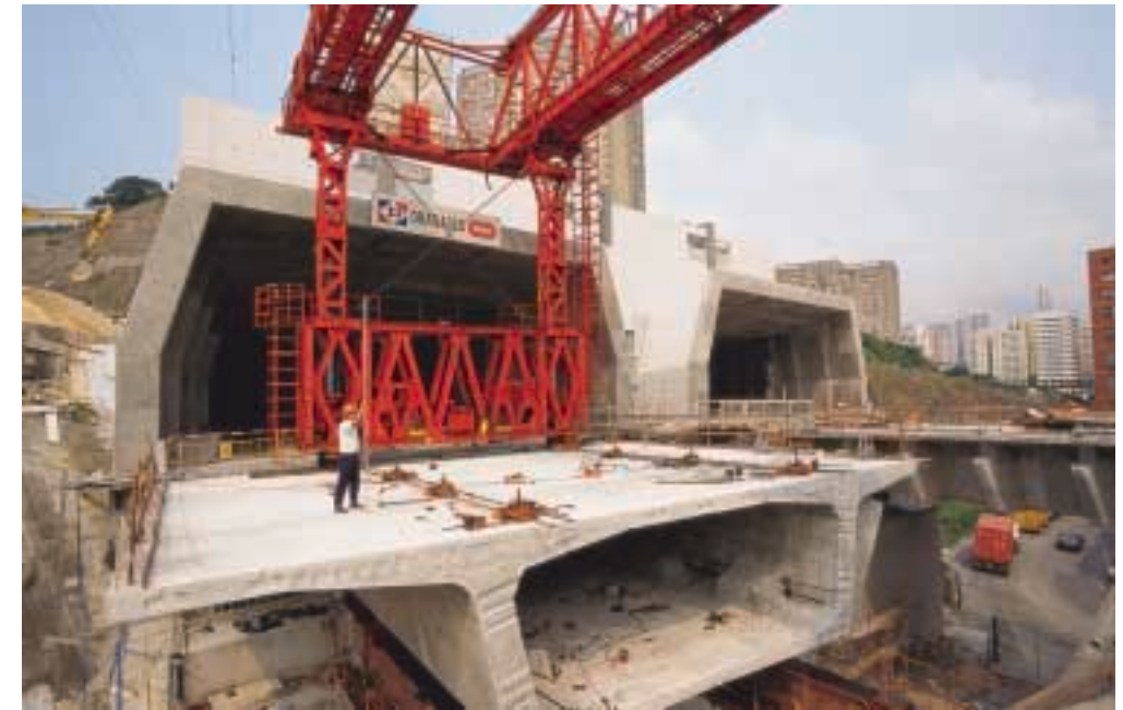
Installing a segment with external prestressing 利用外環預應力安裝組件
