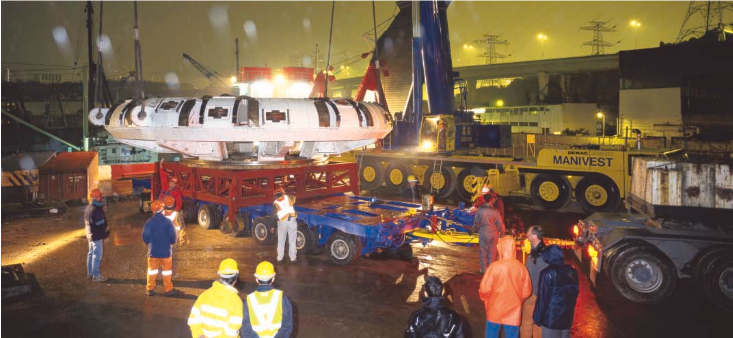
Arrival of the massive TBM cutterhead 隧道鑽挖機的龐大鑽頭送抵工地
