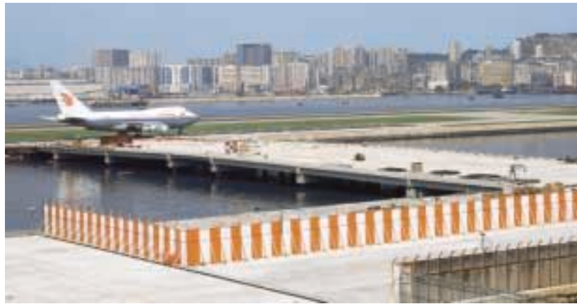
The bridge was built to accommodate two Boeing 747-400Fs 大橋可承受兩架波音 747-400F 型飛機的重量
