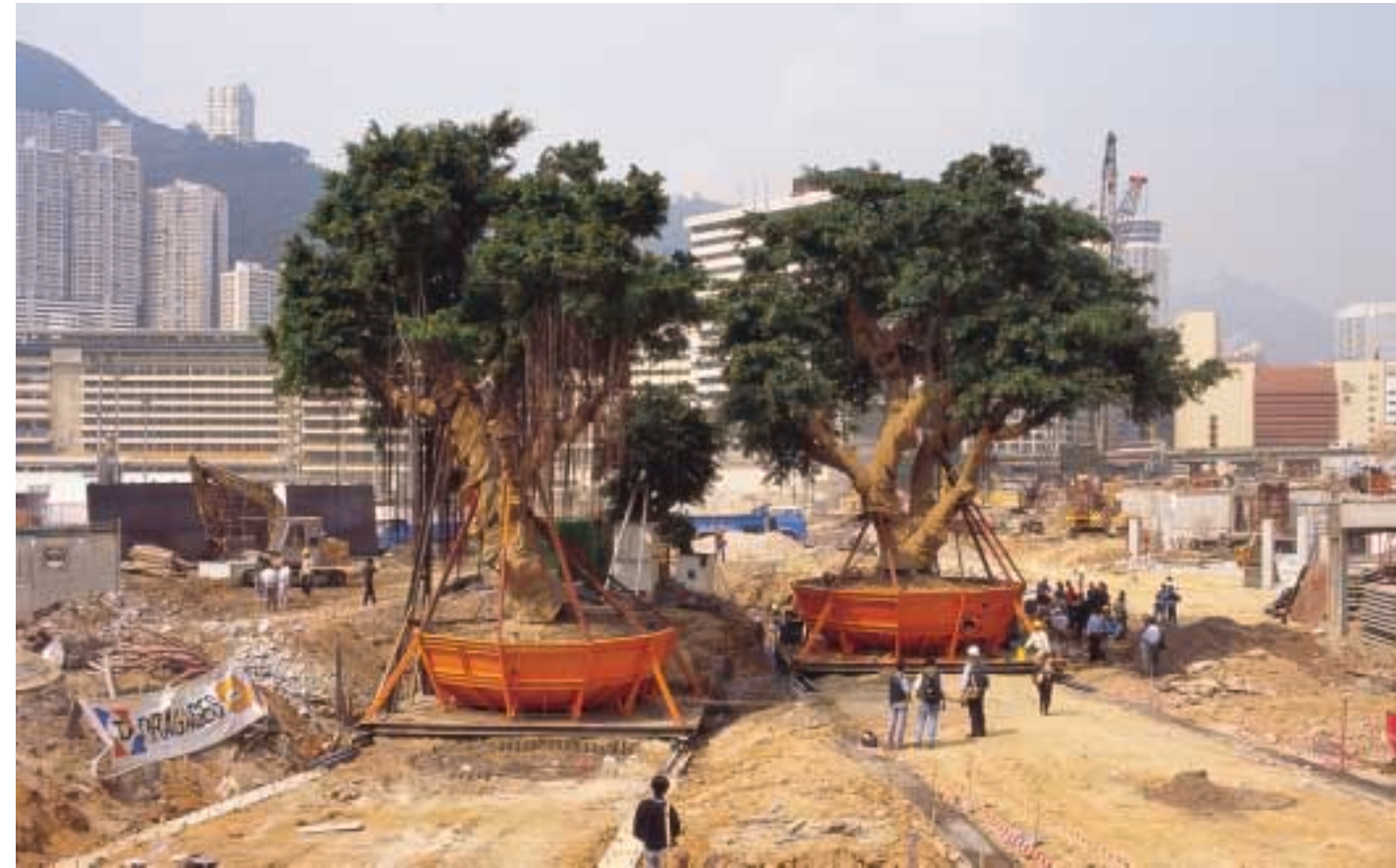
The relocation of two 120-year old trees on special tracks 以特製軌道，輔助移植百年老樹
