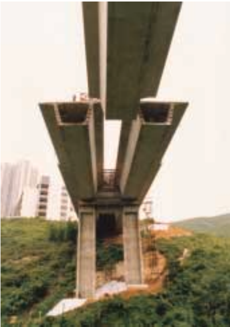
The third box girder was moved carefully into place 安裝第三座箱形大樑
