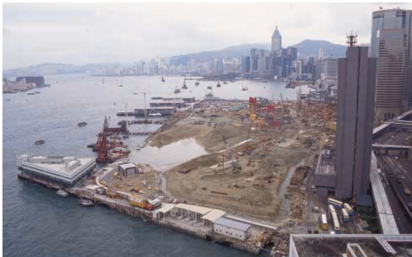
Creating the land within the raised bunds 在土堤之間，開闢土地
