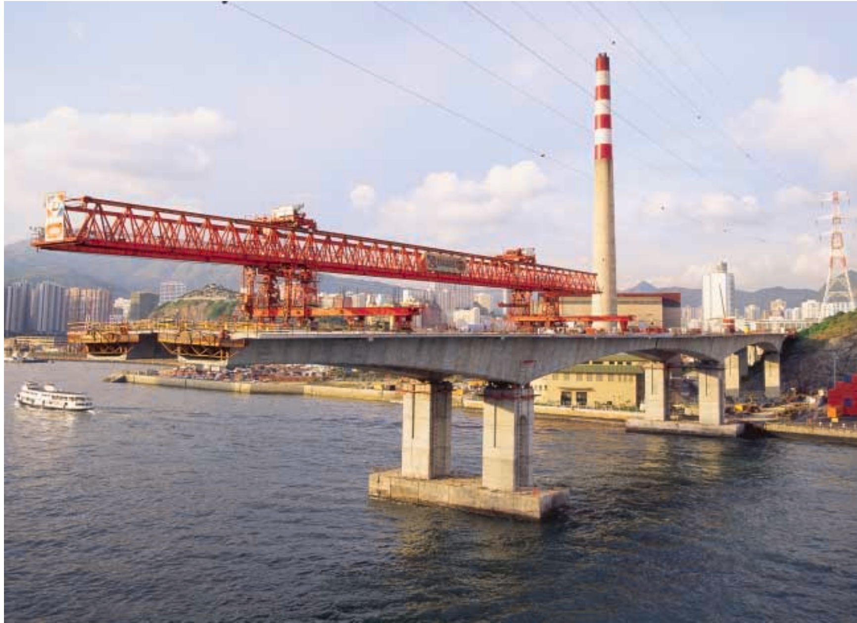
Huge segments were placed without disrupting marine traffic 施工期間，藍巴勒海峽航道保持暢通無阻
