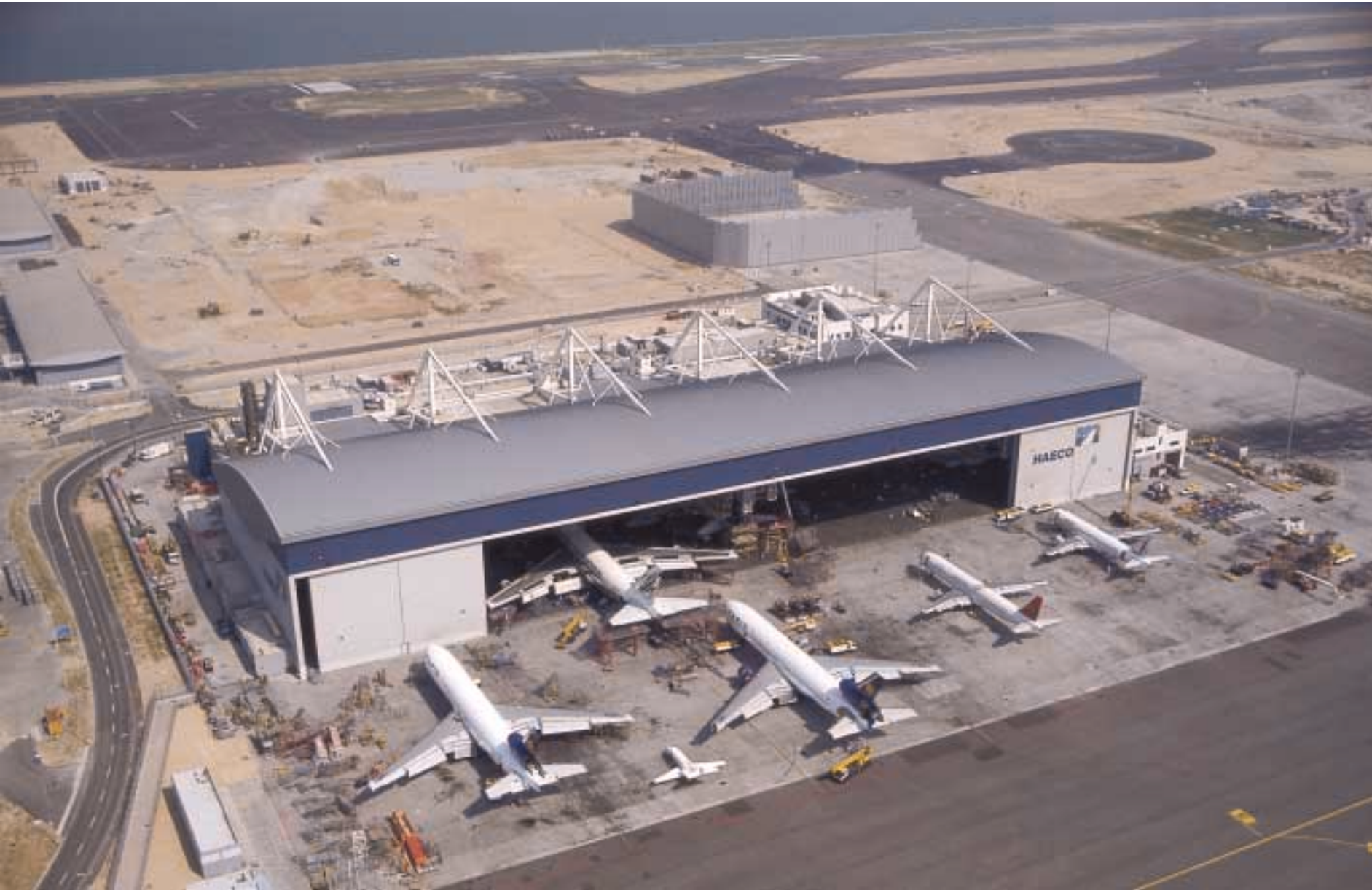
The massive hangar had to accommodate three jumbos side-by-side 無柱式的飛機庫能容納三架珍寶飛機並排停放
