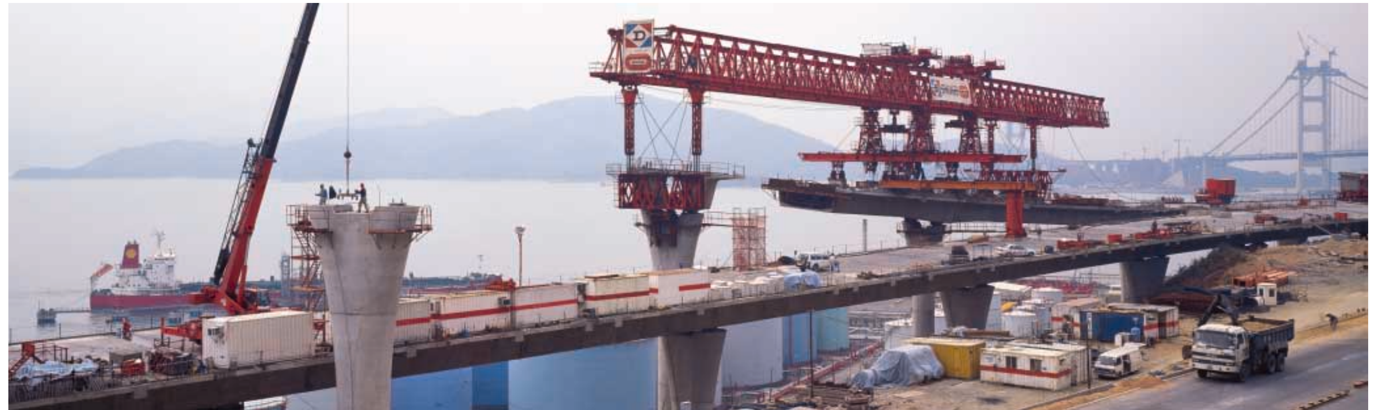
The launching girder placing a massive pier segment 以曳進吊樑機安裝橋樑組件
