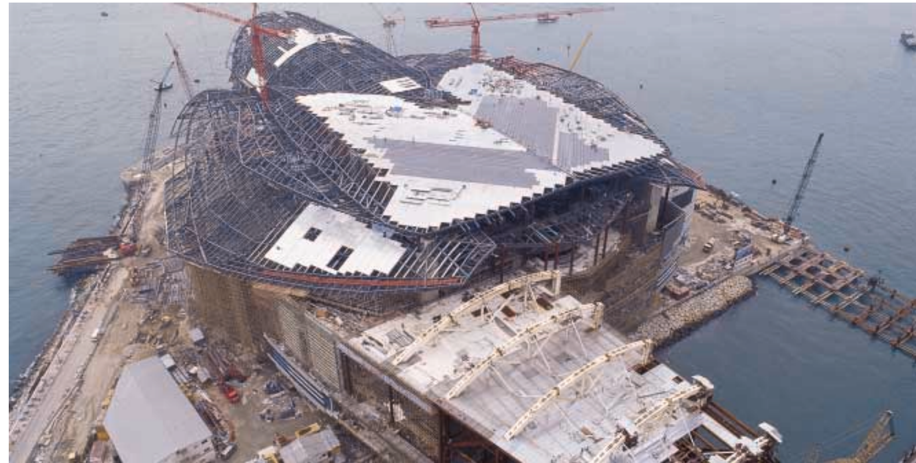
Over 20,000 tonnes of steel were used to build the extension 新翼工程使用逾 20,000 噸鋼鐵
