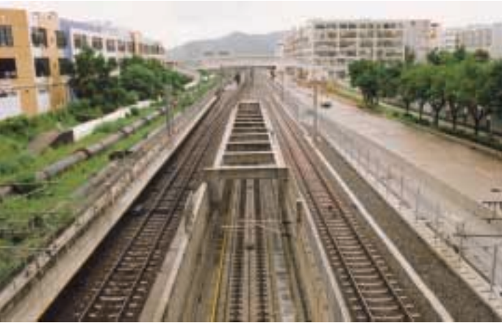
The new rail tracks 新建路軌
