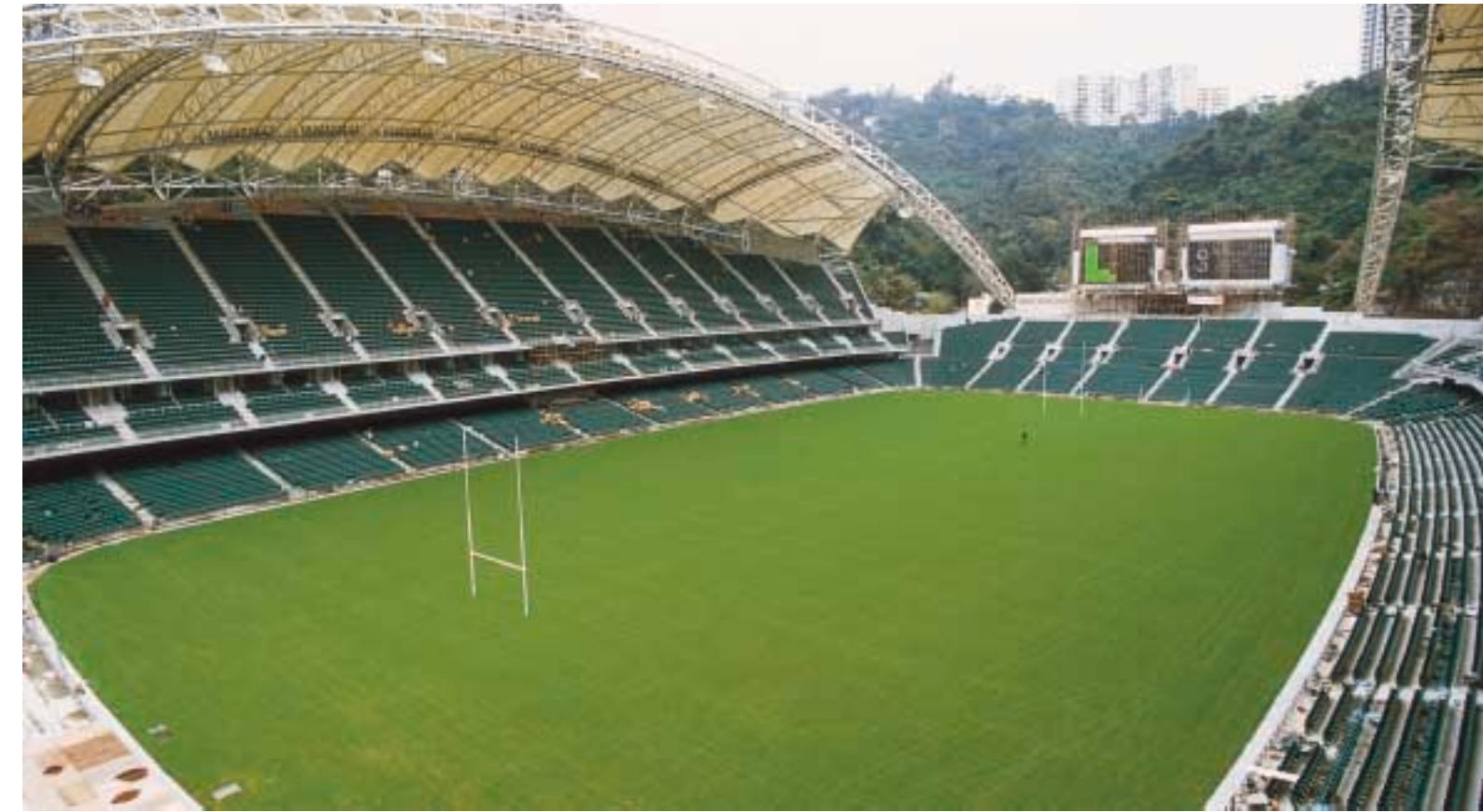
The roof spans more than 240 metres 天幕跨度超過 240 米
