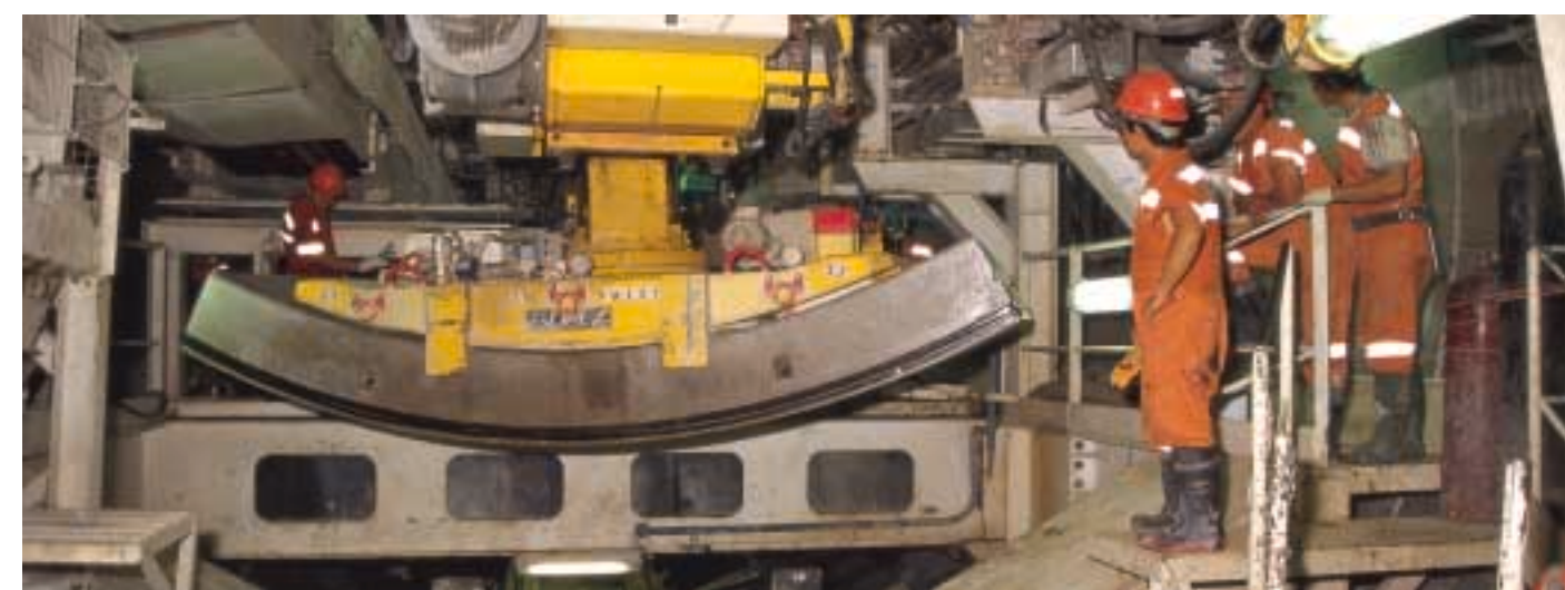
Automatic installation of tunnel segments 自動組裝隧道組件
