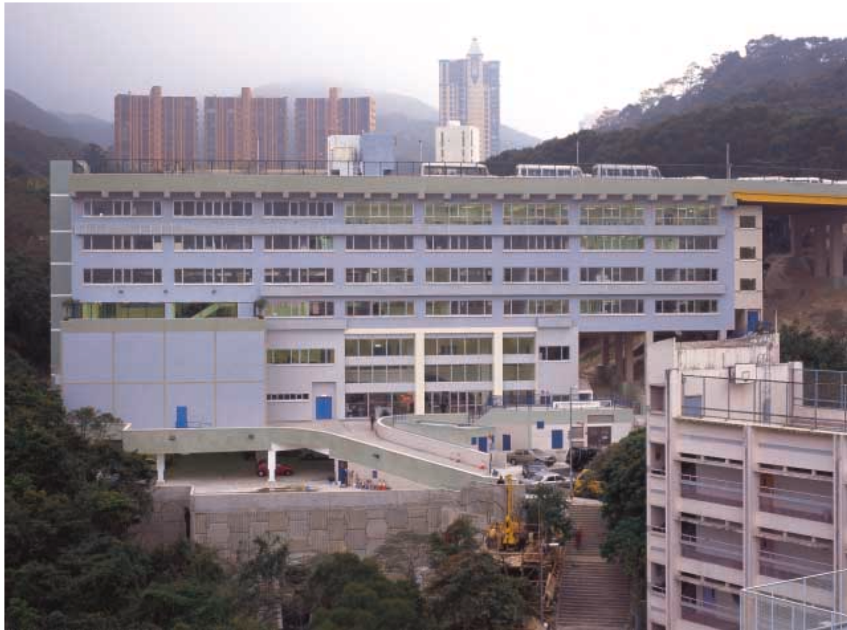
A roof-top bus access platform 建於樓頂的停車坪，方便巴士出入
