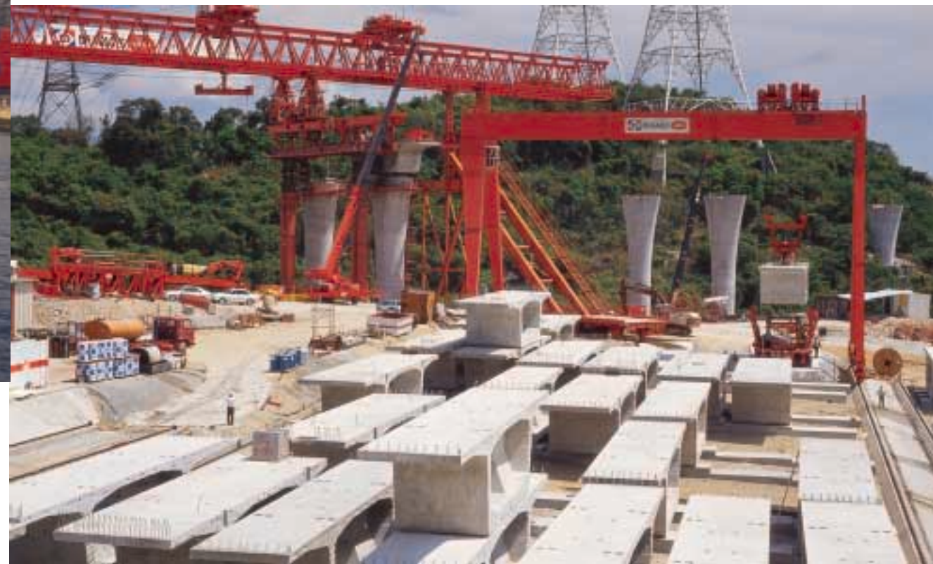
Precast segments being moved to the bridge deck 工程師把預製組件升高至橋面
