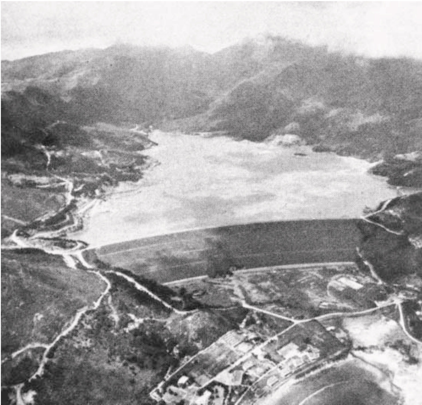
Hong Kong's growing population demands new fresh water supplies 香港人口急速膨脹，急需要開發新水源
