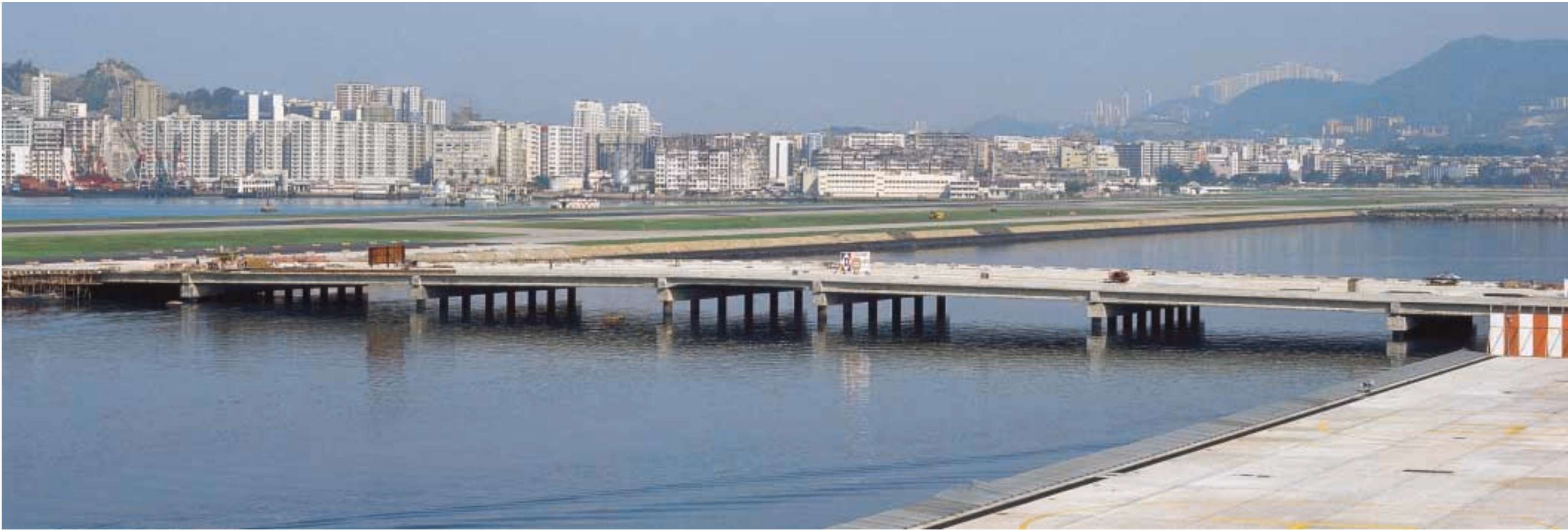
The bridge was built to accommodate two Boeing 747-400Fs 大橋可承受兩架波音 747-400F 型飛機的重量
