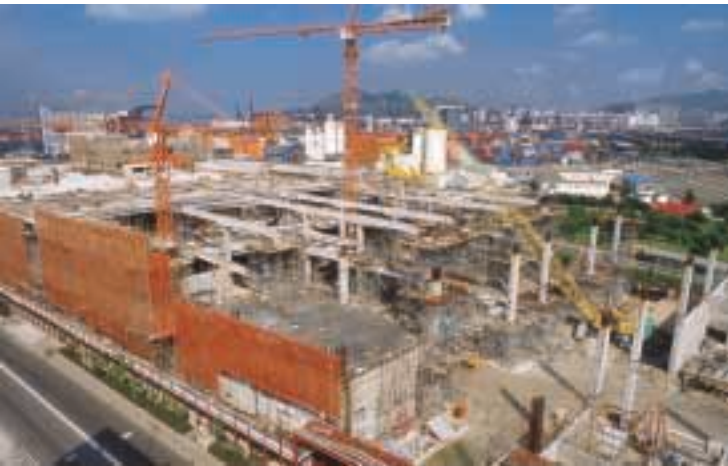
More than 800 precast beams were used 整幢車廠由超過 800 條的預製橫樑支撐
