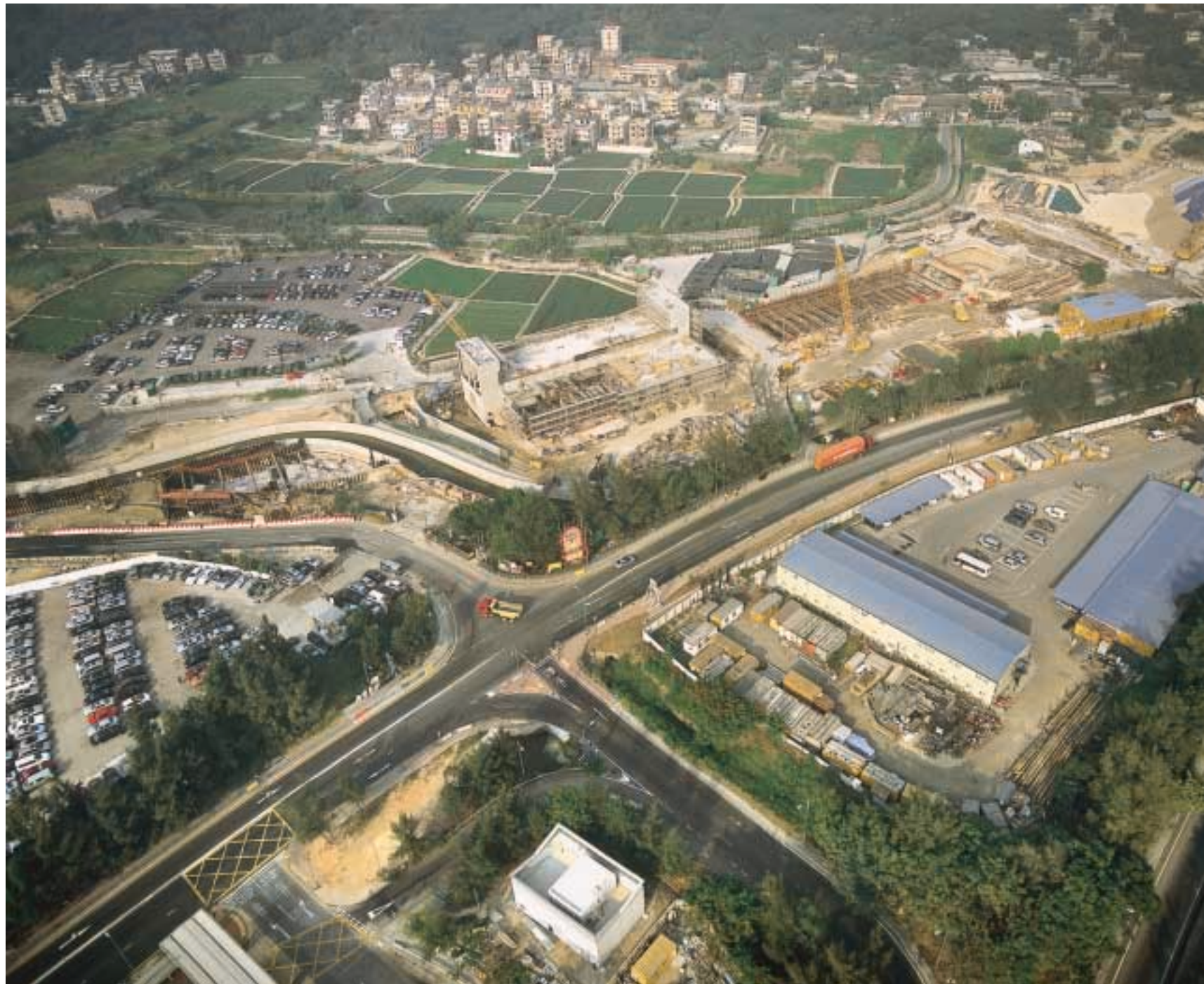
Construction works being carried out among the rice paddies 工程師在稻田之間施工
