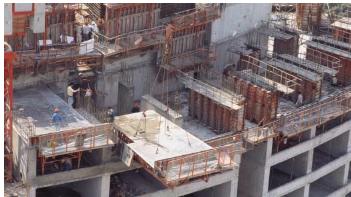
The application of table forms accelerated building works 工程小組以枱模施工，加快工程進度
