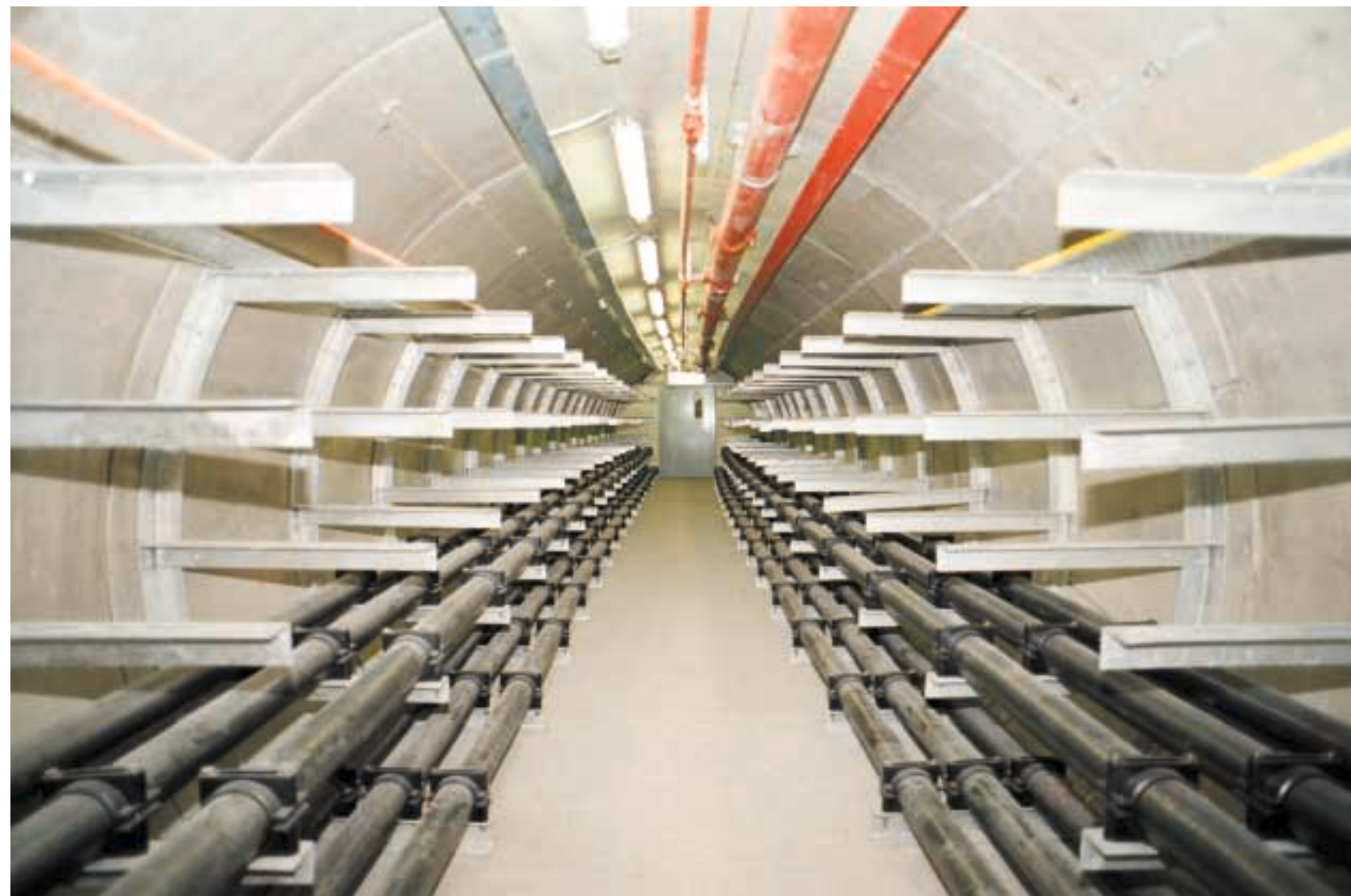
View into a power cable tunnel 電纜隧道內望
