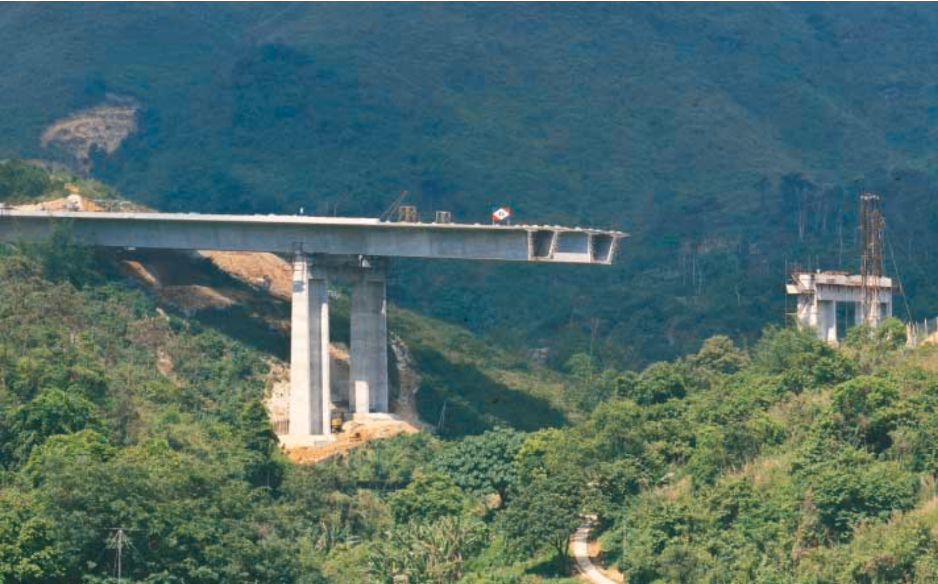
The first and second box girders in their final positions 首兩座箱形大樑就位
