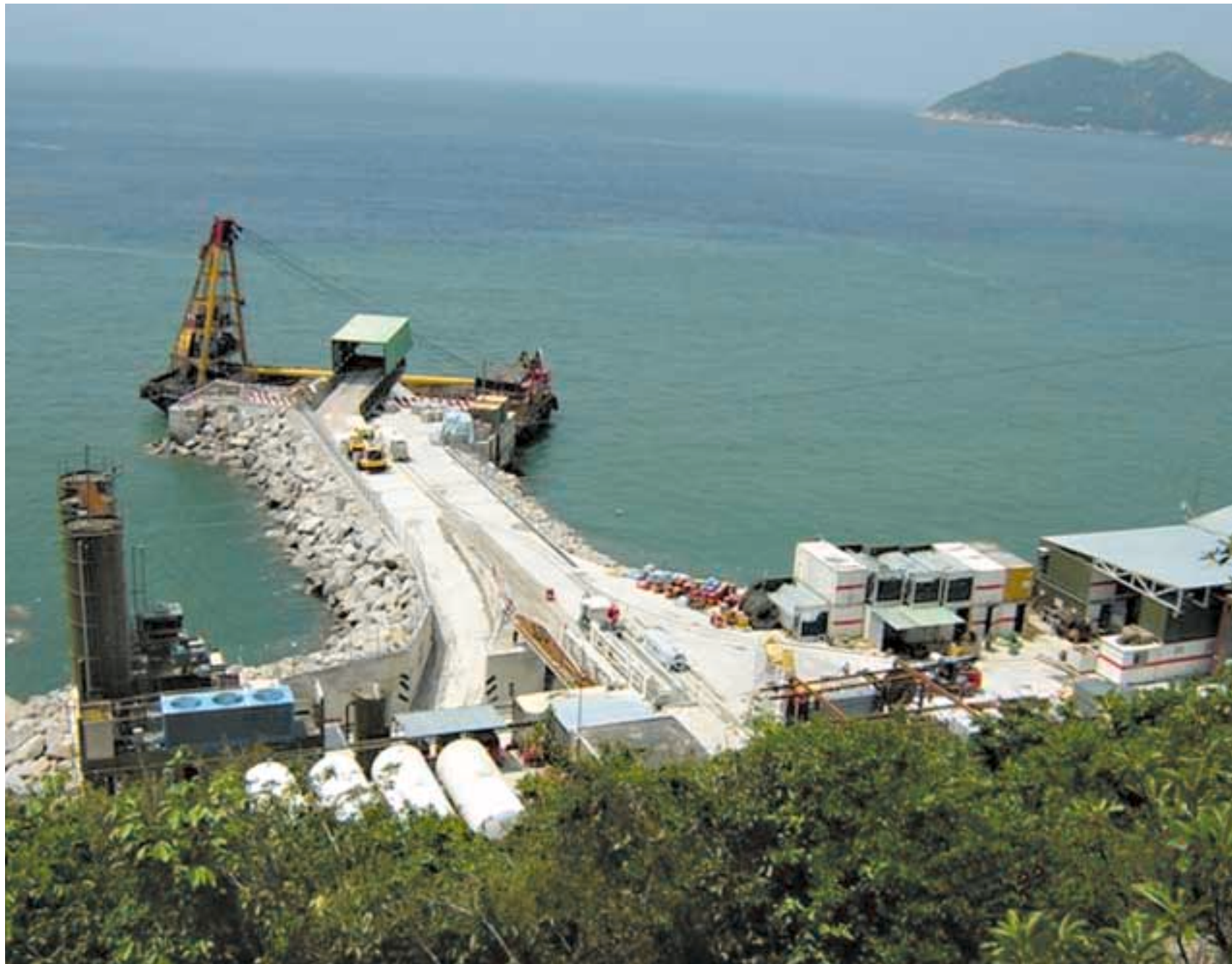
The Chi Ma Wan work site 芝麻灣工地
