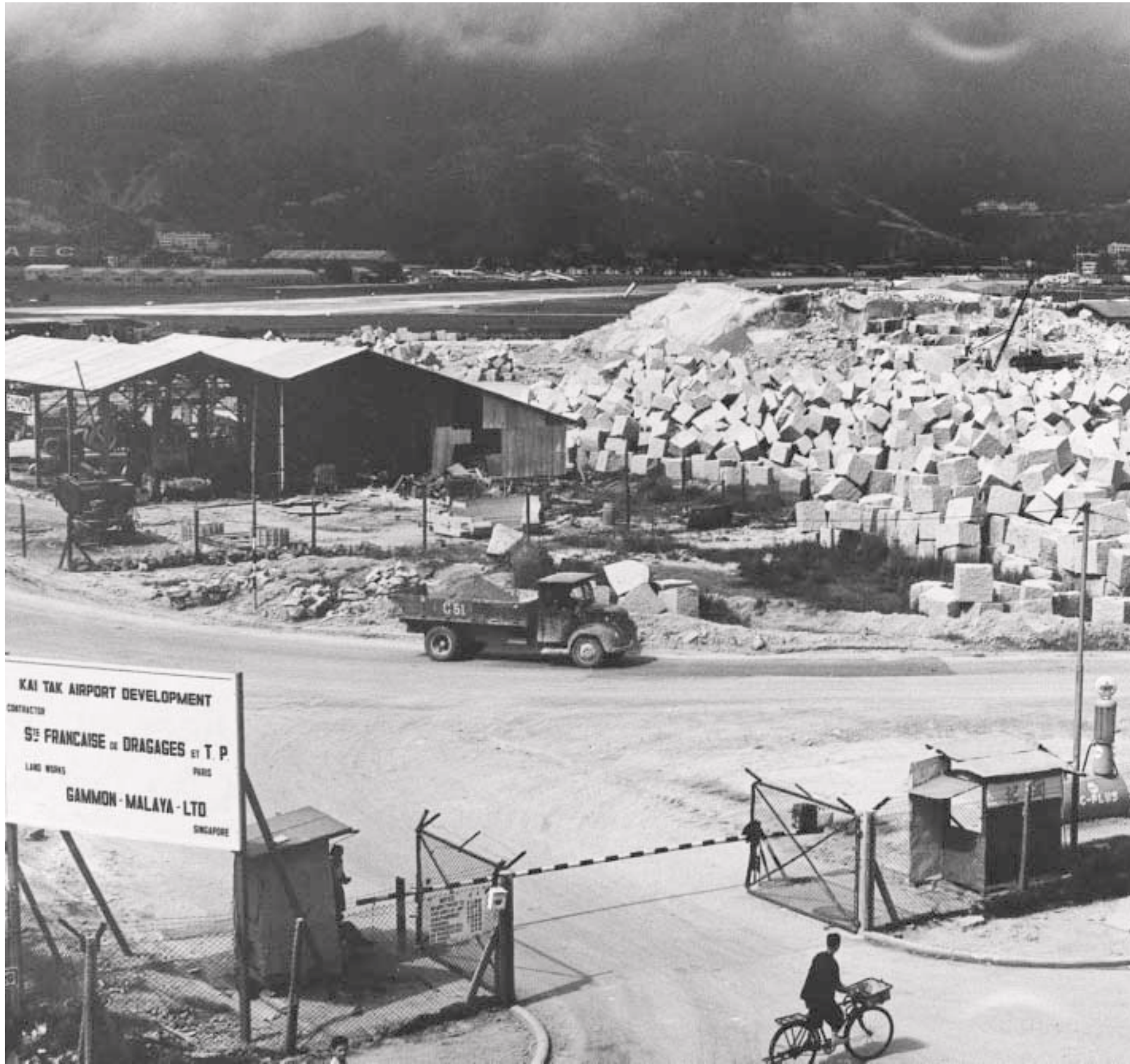
Almost 8,500,000 m 3 of rock was used in the runway 興建跑道需要約 8,500,000 立方米填石
