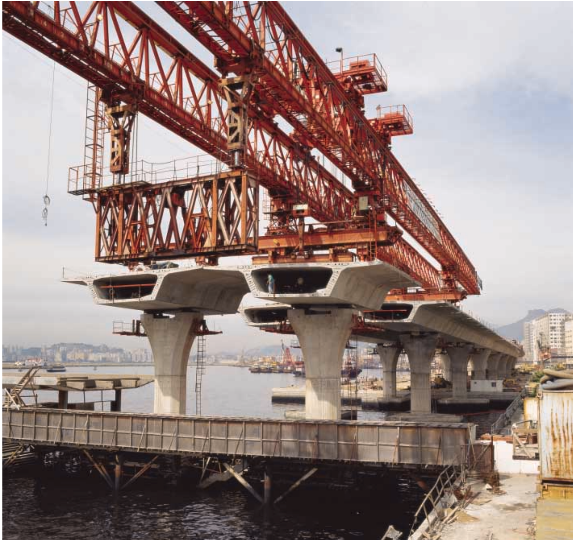
The launching girder was able to place two segments at a time 工程師運用曳進吊樑機，同時間安裝兩段橋樑組件
