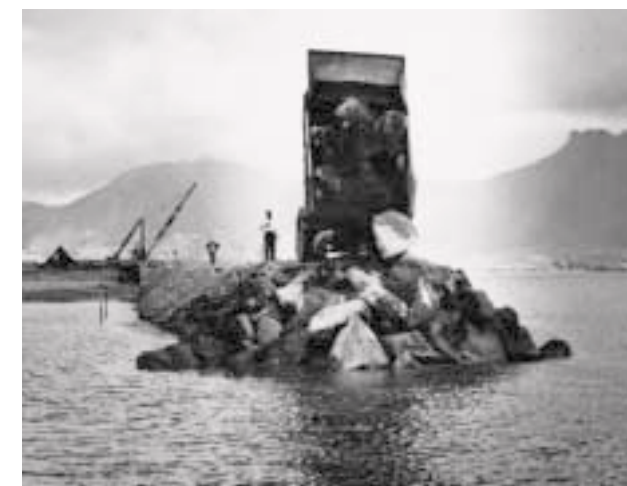
...and placing them into the sea ...傾卸填海
