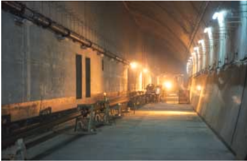
A section of the completed internal partition wall 管道內部間隔牆
