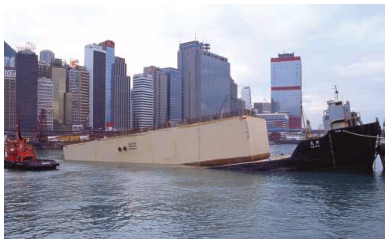
Sinking the tunnel segment into place 隧道沉降至擬定位置
