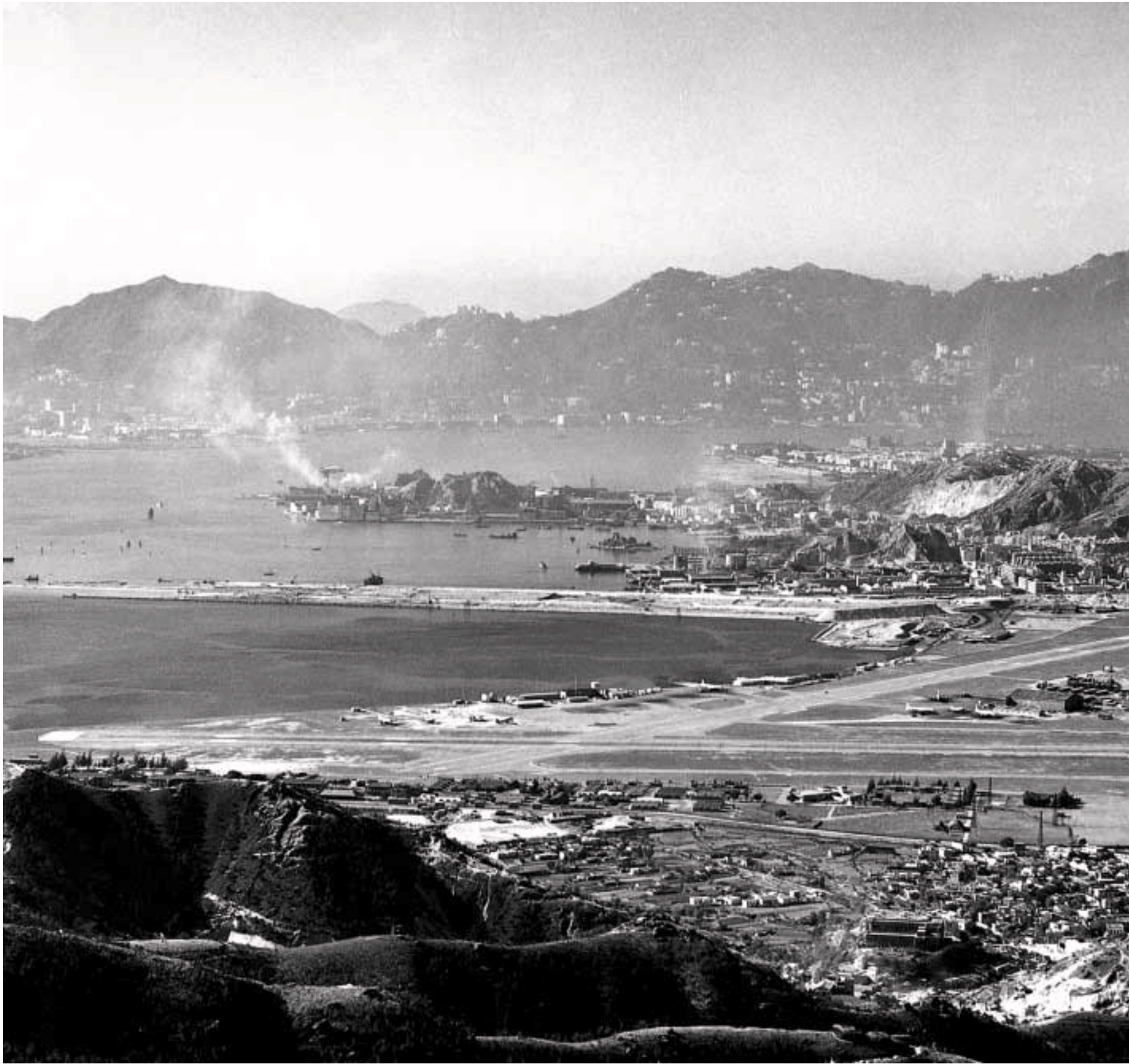
The runway at Hong Kong's Kai Tak Airport was the first of its kind in the world to be constructed over the seabed 香港是世界上首個地方在海床上興建飛機跑道
