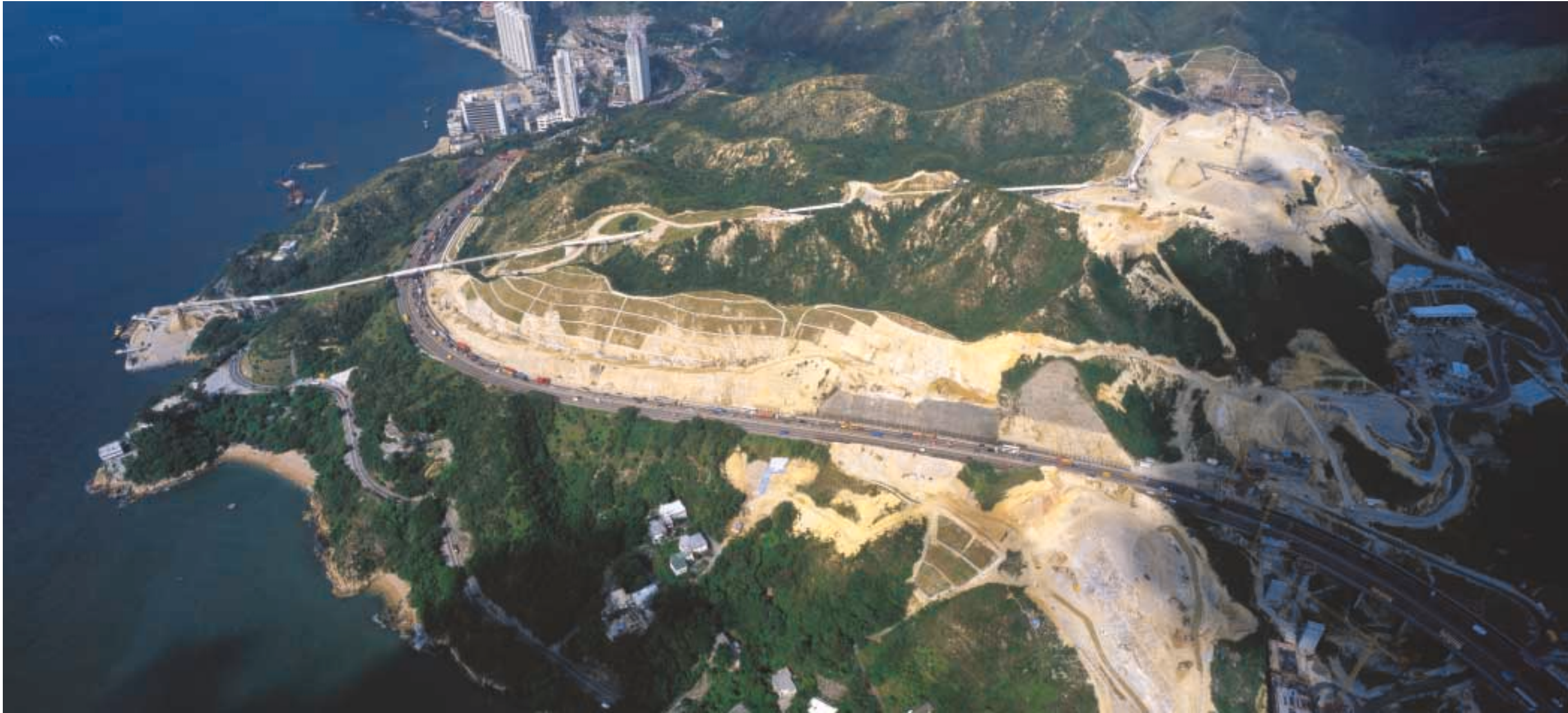
Excavated materials were removed via an extended conveyor system 寶嘉起用輸送帶運送挖掘出來的碎石泥頭
