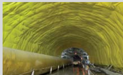
Waterproofing before lining
